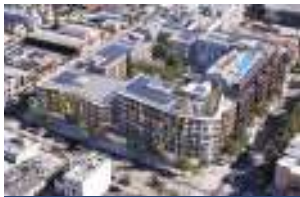
1. 710 Broadway Blvd 280 Units | Compl. 2025
